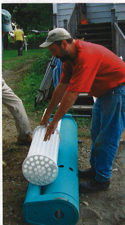
An Orenco Biotube unit is readied for an AdvanTex treatment system.
