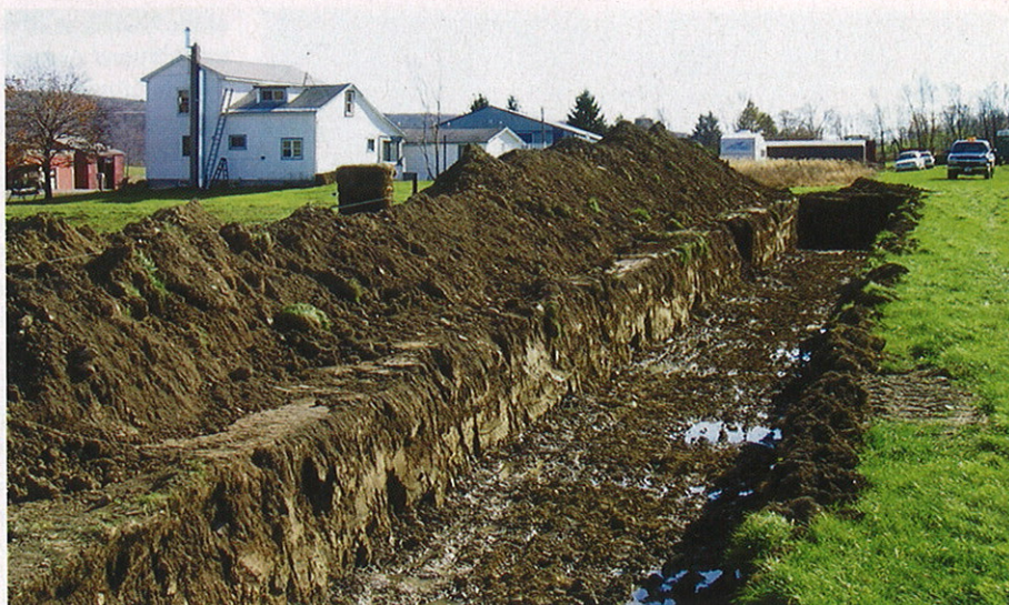
The excavation is made on a cut-and-fill bed for Eljen In-Drains.
