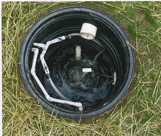
Air bubbles roll in a Knight Treatment Systems White Knight microbial inoculator generator.
