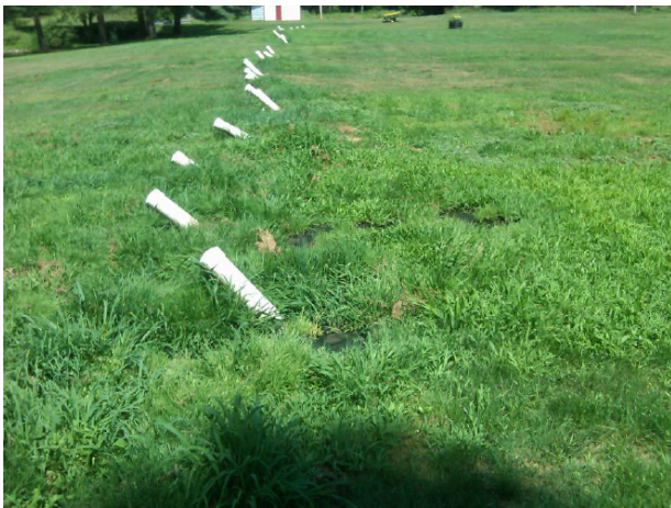
Before (Flooded with wastewater)
