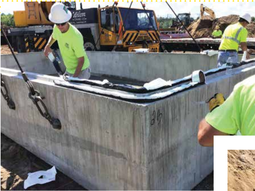
◀ Thomas Fiacco III (left) and Peter Arcadi from TJ Fiacco Construction apply butyl rope sealant to the bottom half of Tank 5. Barry Cook is in the background.
